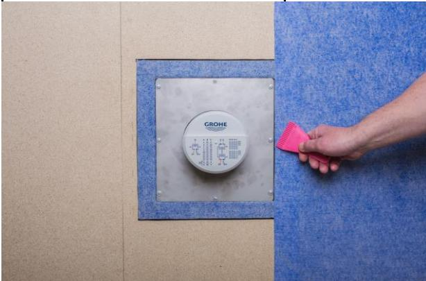
4 - Seal the seam between the wall foil and the prefabricated foil flange using GKHero pro wet room membrane. (2 layers)
